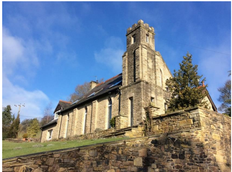
2 Converted chapel in Mill Brow
